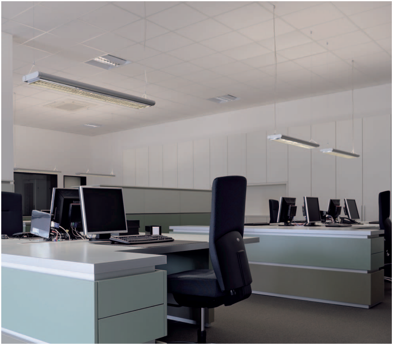
The pendant luminaires Long Grill and Work light are equipped with a Dark-Light grid, suitable for display work stations according to DIN 5035-7. This allows an optimal illuminated work station and glare free light.
